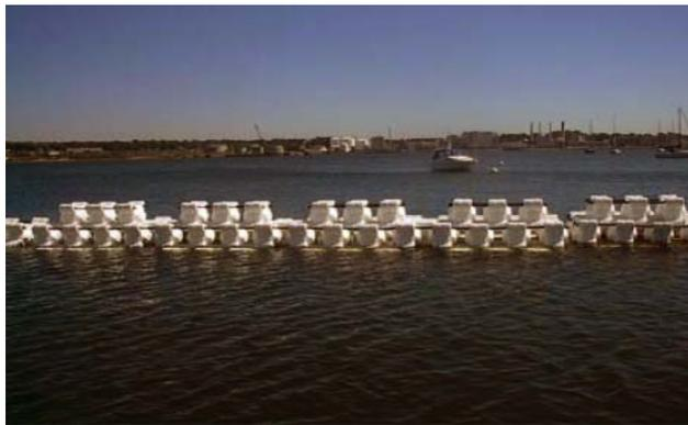
Marina on Sodus Bay in Lake Ontario, New York we are showing a transmission coefficient of 0.1 on the expected wave spectrum. The Marine Barrier was able to dissipate the 4foot waves that the marina was subject to during highly destructive storms to a mere 6 inches (90% efficient)!
